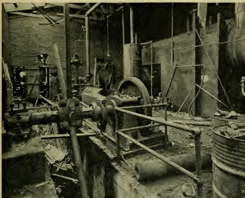
Engine room after the shattering of the flywheel. All that remains of the wheel is the hub and three spokes.
